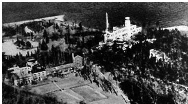
main house and powerhouse smokestack, upper right; service buildings, lower left
